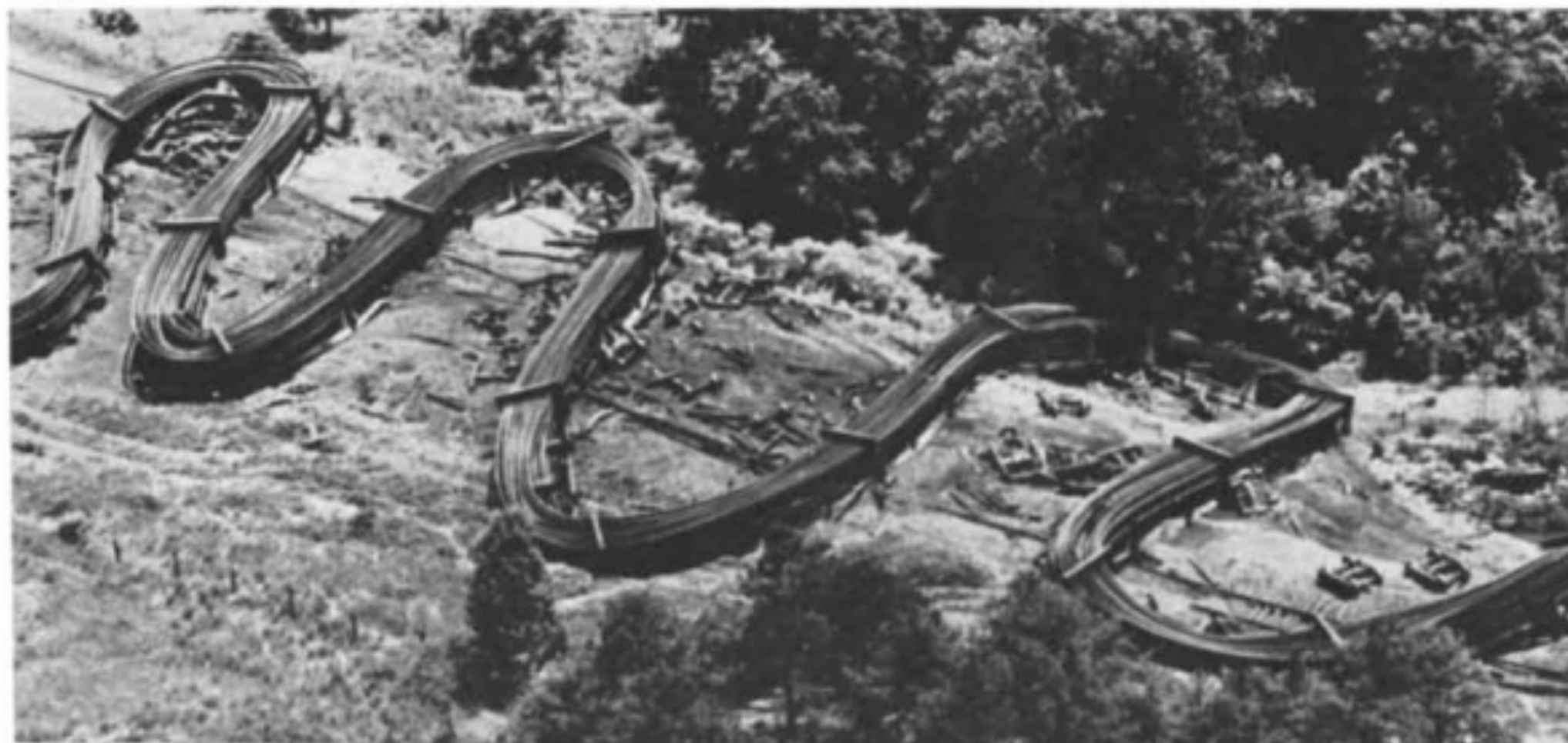
CATASTROPHIC EXAMPLE of the potential consequences of a weak design. The bridge design folded the critical load path into a
